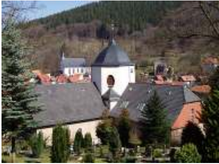
View to the church from south-west
